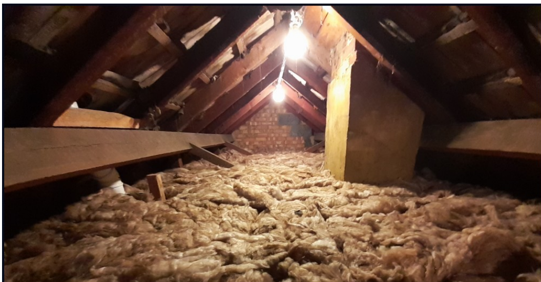
The finished insulation system
