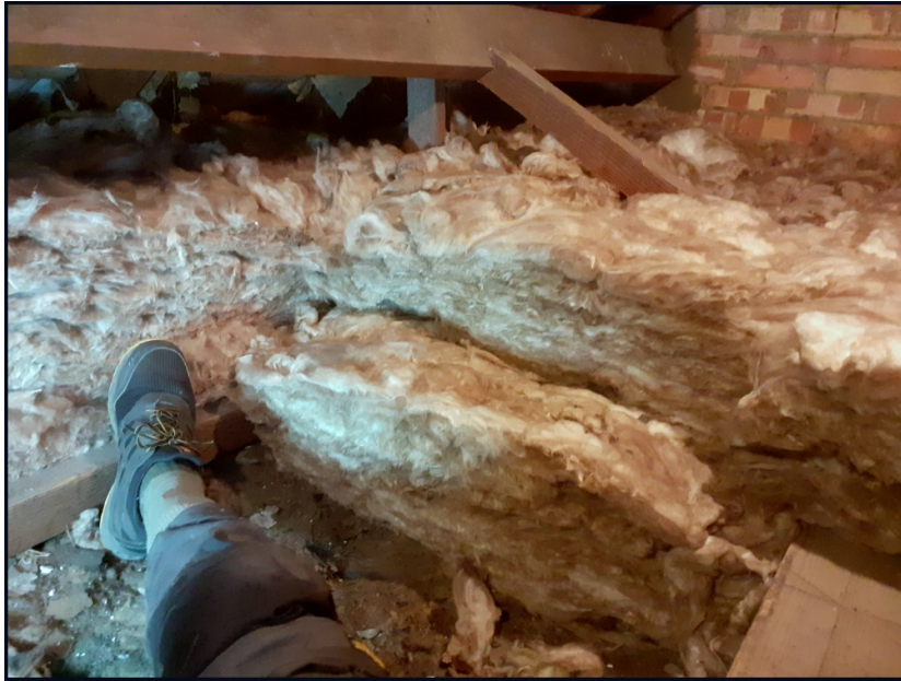
Image showing the two layers of 200mm glass wool
